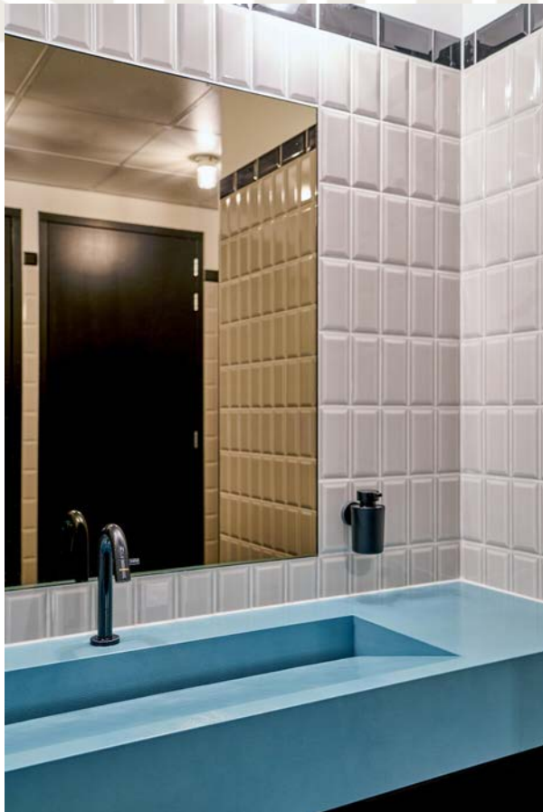
In the toilet areas the wall-filling sinks stand out. Functional and beautifully executed, cast in one piece in colored epoxy.
